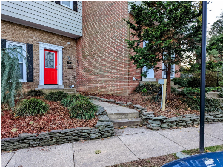
EV charging outlet in Monet Dr, Rockville townhome community
